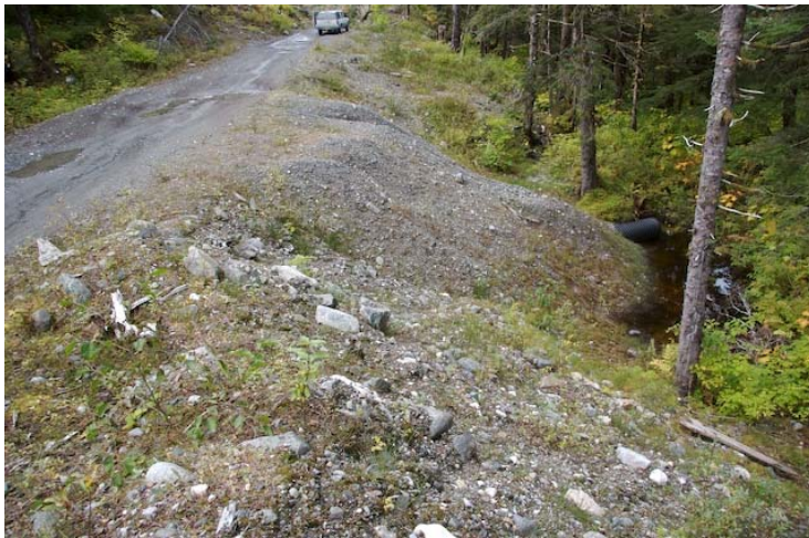
Photo 3: Erosion on inland subdivision road, September 2007.
