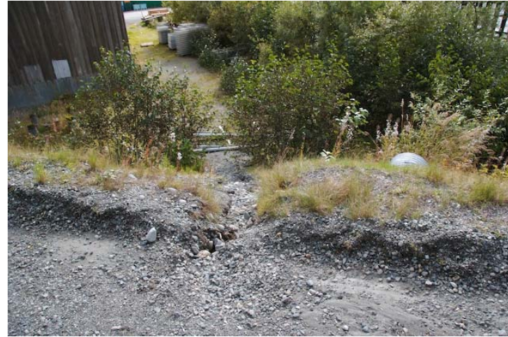
Photo 2: Erosion by Ocean Dock, September 2007.
