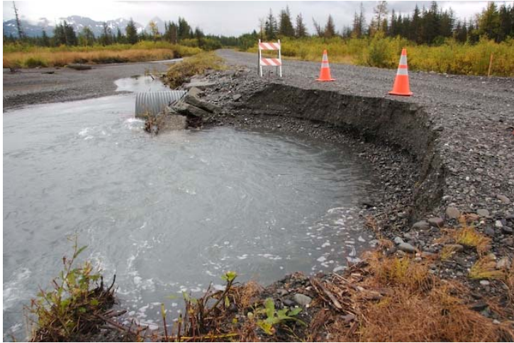
Photo 1: Erosion on Forest Highway, September 2007.
