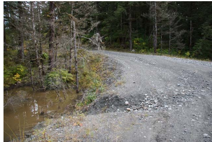
Photo 4: Erosion on inland subdivision road, September 2007.
